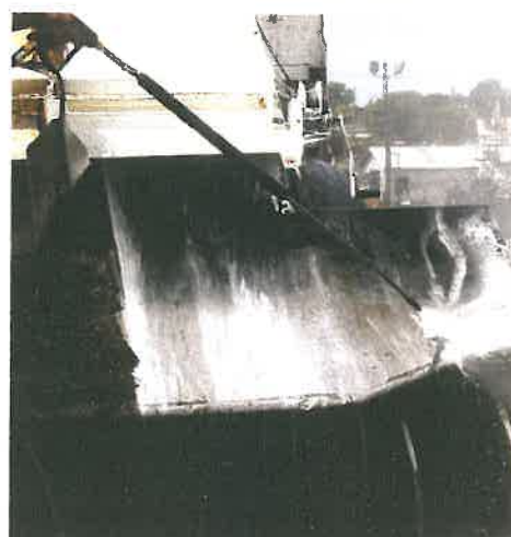
Flush with Water Pressure
