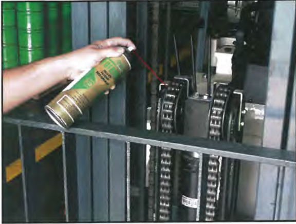
OPEN GEAR LUBRICATION
