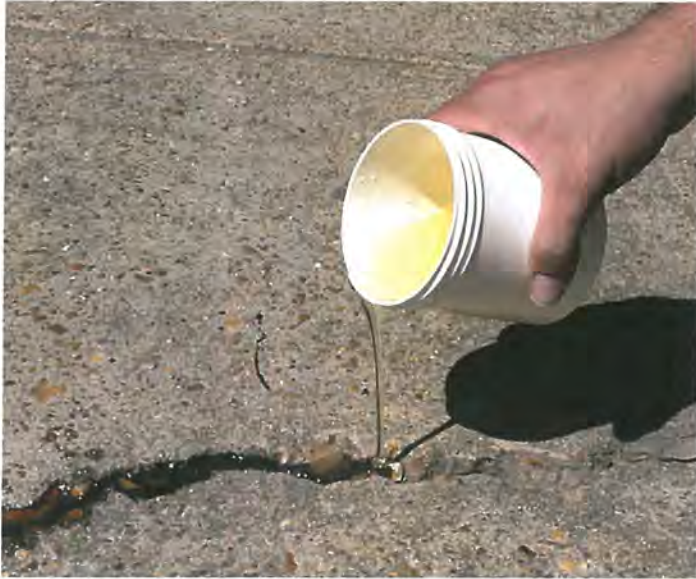
Repairs Joints In Concrete Floors
