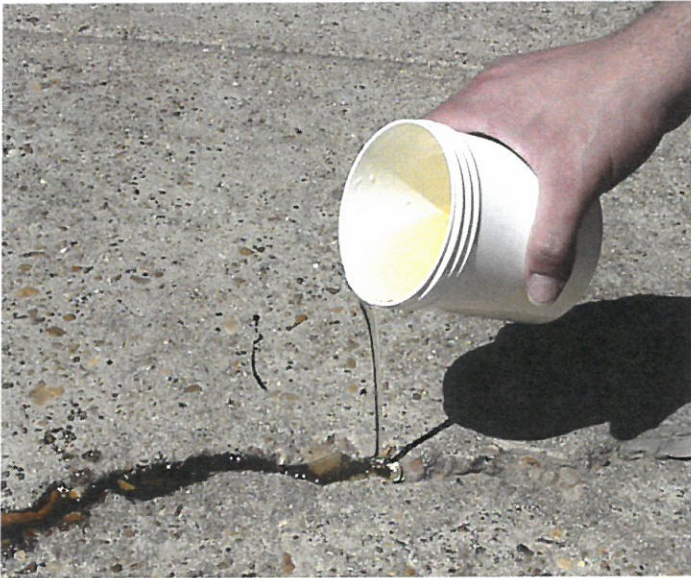
Repairs Joints In Concrete Floors
